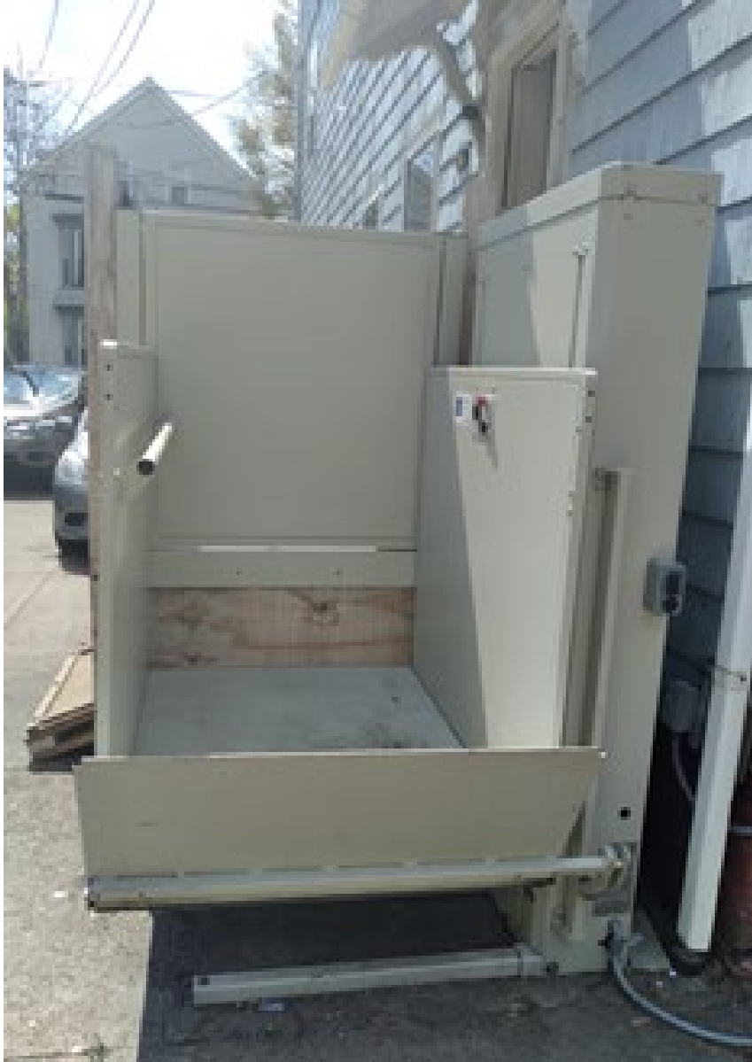
A new deck and vertical platform lift were installed.
