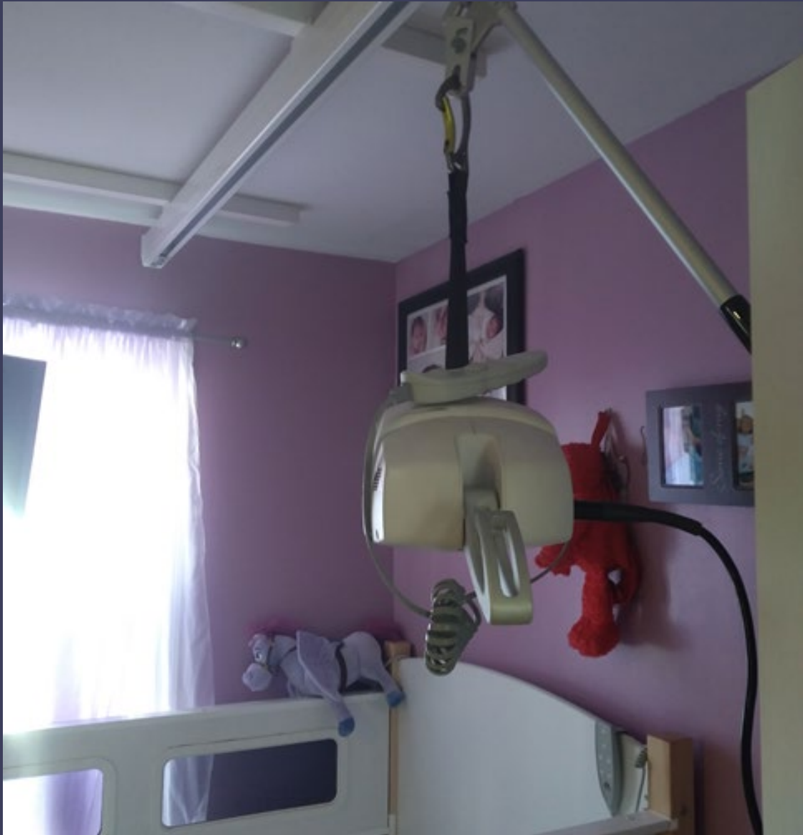
A ceiling lift was installed over the bed.
